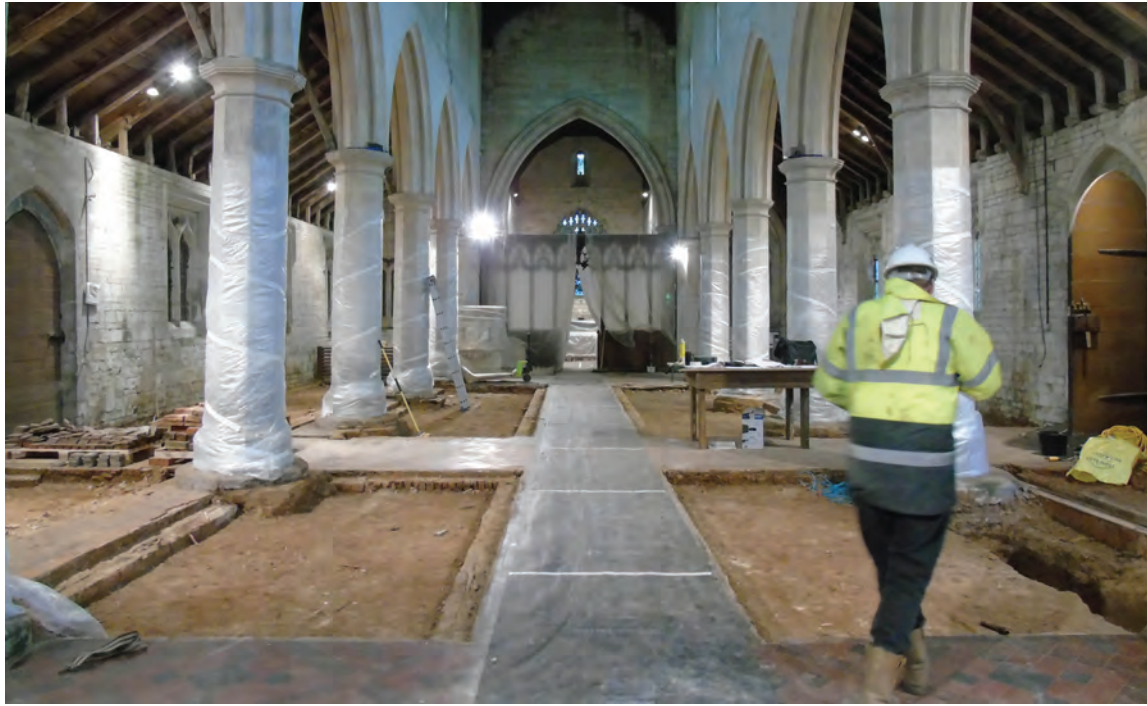
Above: All Saints' Church, Benington, under construction
